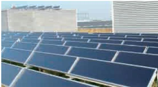
The TiNOX absorbers are energy traps. They collect almost all available solar radiation and convert **The energy trap** it into heat. Unlike black chrome or black-coated absorbers, almost none of this energy is lost again as heat radiation. The energy is directly transferred into the heating-support and water heating systems by the TiNOX absorbers.
